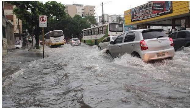
Figure 1: Flooded route after rain in Belém Source: Roma News (2019)
